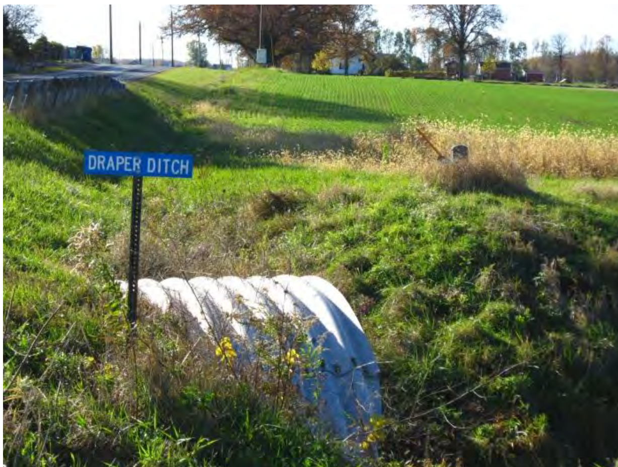
Figure 32: Culverted stream, Draper Ditch. (Christina Znidarsic)
